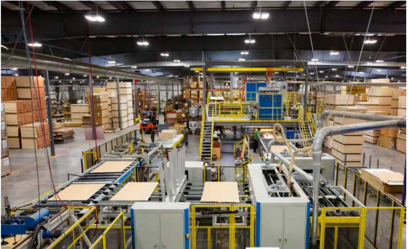
This U-shaped lamination cell line produces “thousands and thousands” of laminated panels for Genesis’ high-volume customers.
